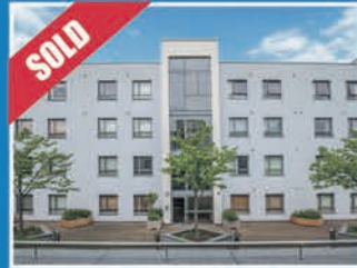
Grove Court Blanchardstown
