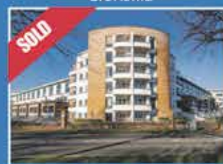
Scariff Hall, Blanchardstown
