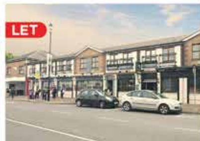
Restaurant, Main St, Blanchardstown
